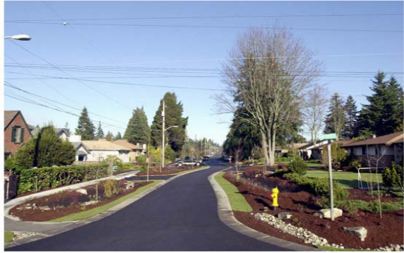
After Completion - January 2001
