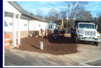
Fine Grading Topsoil
