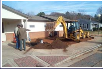
Spreading Amended Soil
