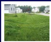
Waterford, CT 2003 BMP Subdivision, Jordan Cove Urban Watershed Project
