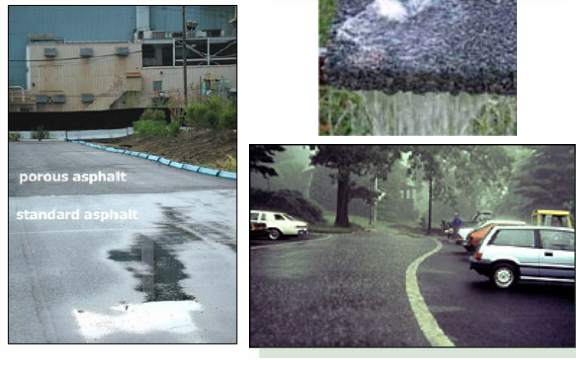
Figure 8-15. Drainage in Both Types of Pavement
