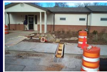
Runnel Installation
