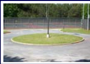
Adjacent Intramural Parking Area (standard curb & gutter island)
