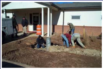
Install River Rock Swale / Cut Overflow
